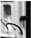
remove four screws and the small cover, feed your supply lines in through the conduit nipple and wire-nut the electric supply wires to the three pigtails already in the junction box. (Four or five wires if three phase).
